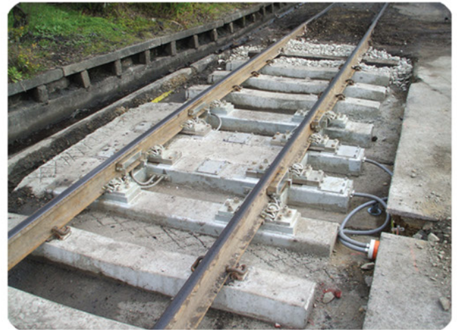
Installing the T-WIM train scale in concrete
