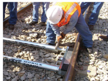
Inserting the MTW into the track
