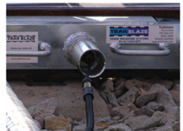
Connecting the cables
