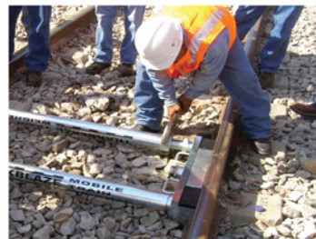
Inserting the PTW-S into the track
