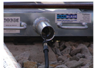
Connecting the cables
