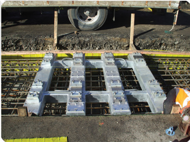
Installing the T-WIM train scale in concrete
